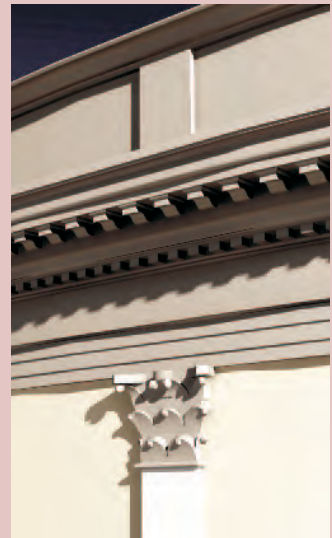
Fig. 93 – Reconstruction of the decoration of the upper section of the theatre's exterior wall. Corinthian pilasters supported a cornice surmounted by an attic.
