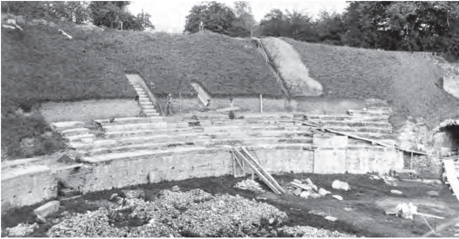
Fig. 52 – Amphitheatre. View of the reconstruction in 1950 of a section of the tiered seating funded by the patron Maurice Burrus.
