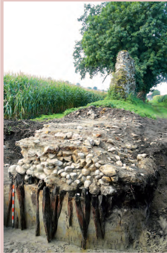
Fig. 117 – City wall. Section of the base of the wall. Oak posts driven into the sandy wet substratum stabilised the stone foundation.
