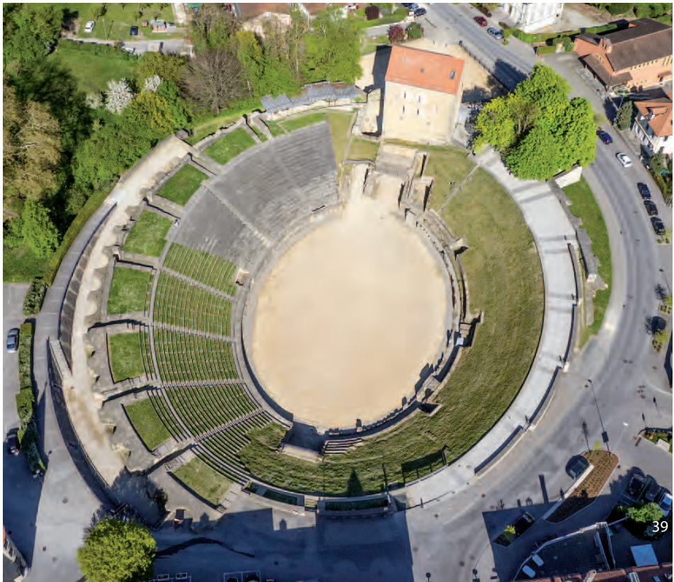
Fig. 47 – Amphitheatre. Aerial photograph (2014) showing the rebuilt tiered seating section and the medieval feature called the «Bishop's Tower» (above the arena's gateway) that houses the Roman Museum.
