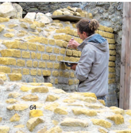
Fig. 88 – A facing of a wall of the theatre under restoration in 2013 with new yellow limestone blocks.
