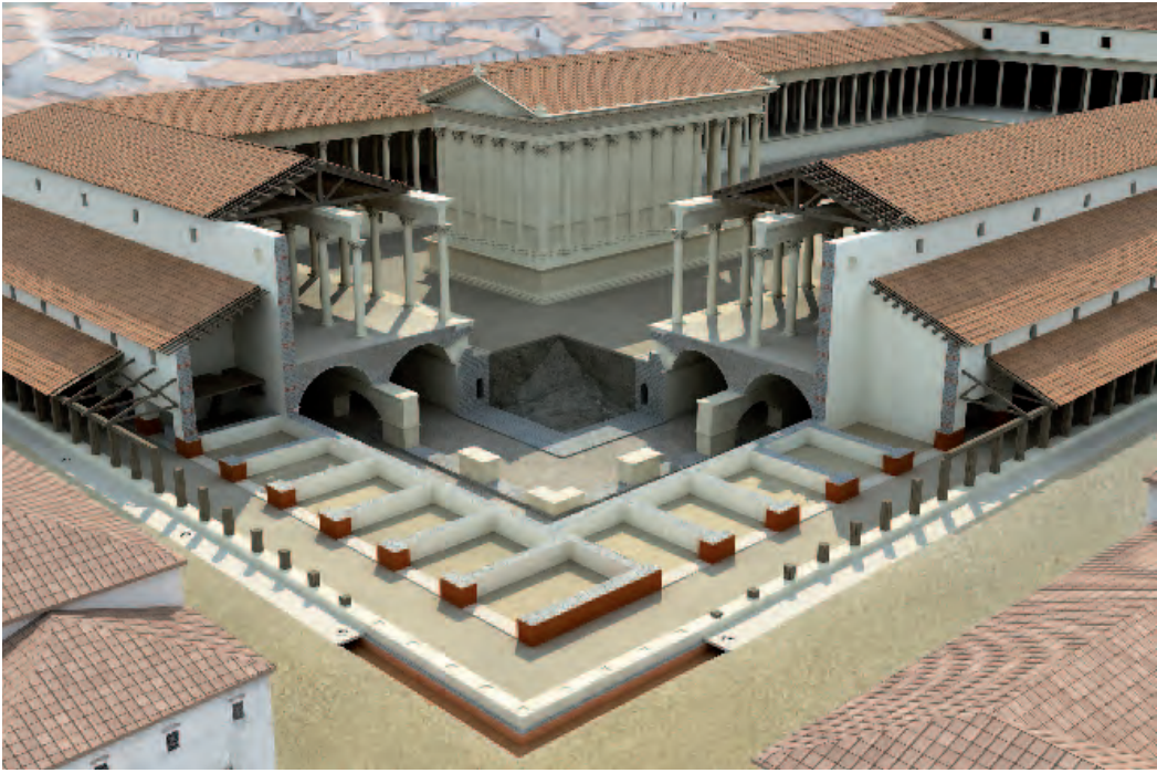
Fig. 98 – Computer assisted model of the Forum of the Roman city of Lutetia (Paris) that was similar to that of Aventicum. The sacred area, viewed from behind, comprised a temple on a podium surrounded by a colonnaded portico above an underground corridor with two naves ( cryptoporticus ). Outside the Forum, were shops facing the streets and preceded by porticoes. Top right, the public area and the Basilica.
