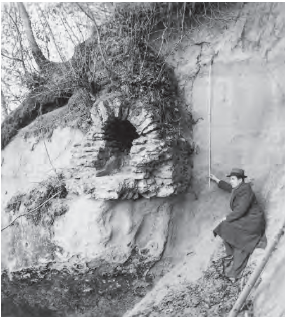
Fig. 167 – View of the section of the underground aqueduct of Coppet. The conduit was cut through the molasse (sandstone) substrate (1941).
